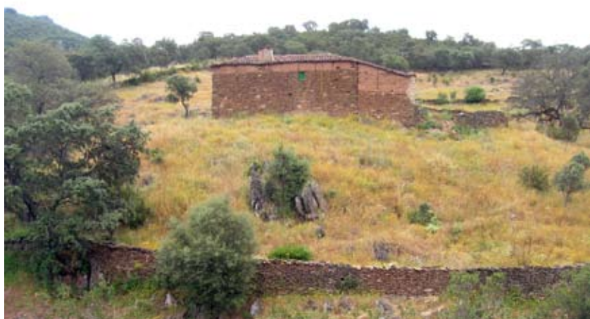
Local architecture features still prevail in some isolated buildings
