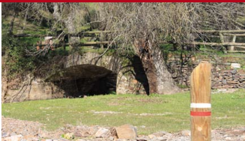
Bridge over La Campana River
